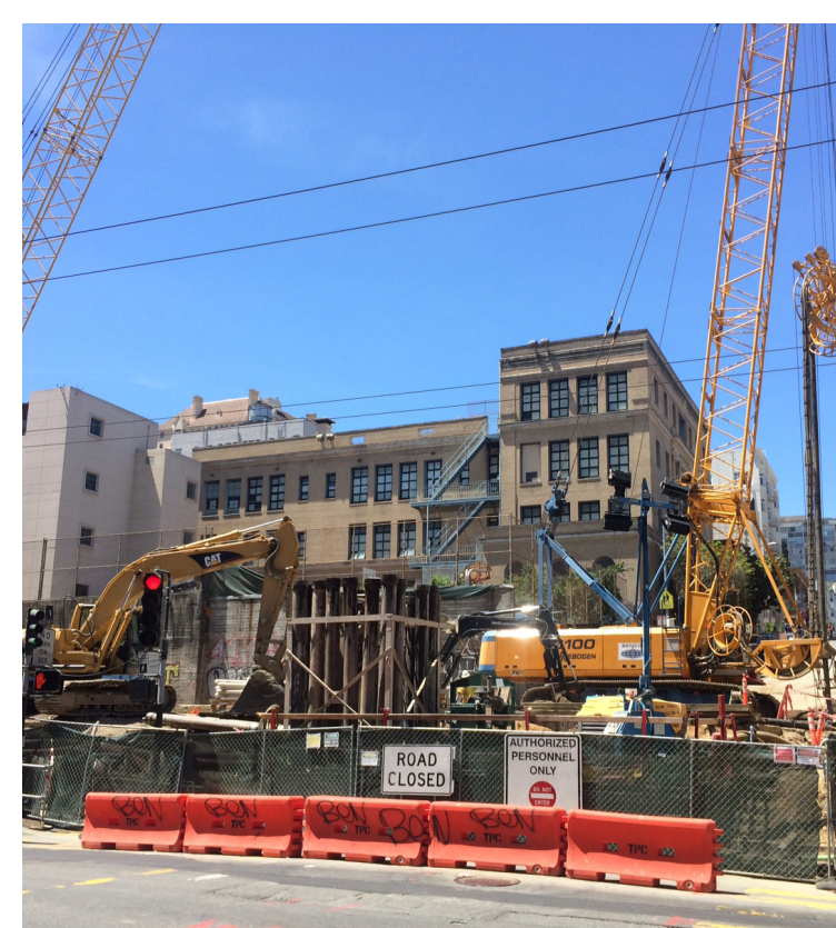
CONSTRUCTION Slurry Wall Construction at the Station
